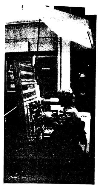
Fig. 12 The 11B system. Sitting posture when working on the lower rows of the frame. Note low-luminance lighting and new chair
